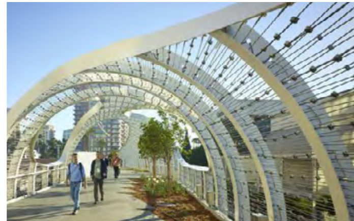
02 Footbridge (Rainbow bridge, USA)
